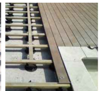
Timber decking on pedestal system
